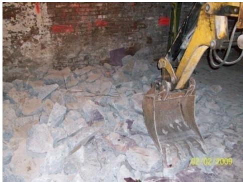
Figure 2: Shows an Excavator in the Demolition Phase
