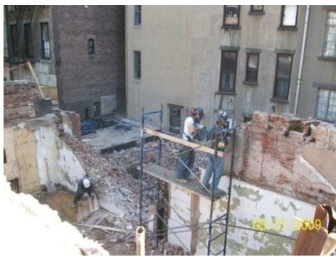
Figure 3: Shows Hand Demolition method being utilized
