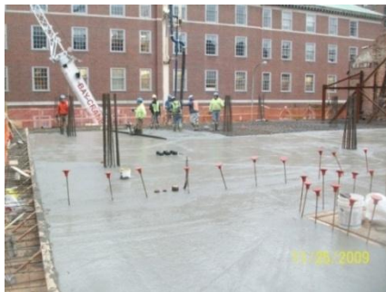
Figure 6: Pump Truck Placement Method
