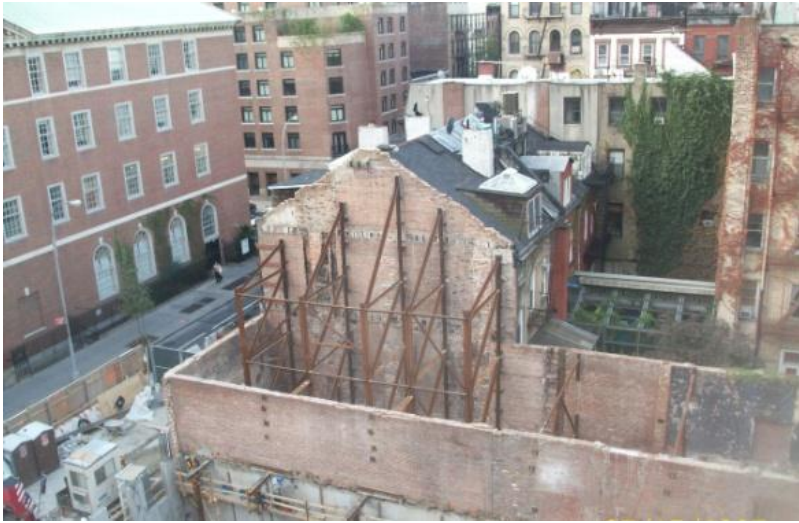
Figure 4: Shows Temporary Structural Steel Bracing
