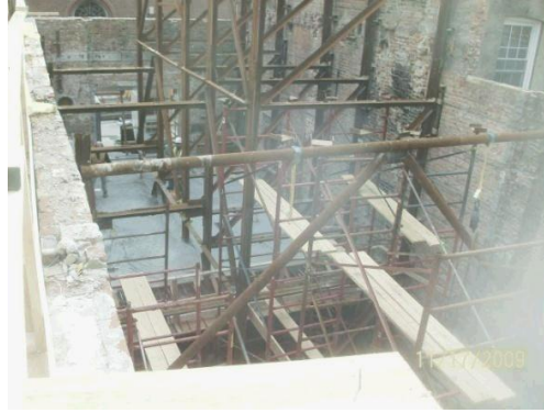
Figure 25: Shows an Up-close View of the Structural Steel Bracing
