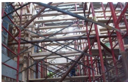
Figure 7: Shows the Addition of Shoring to the Steel Bracing
