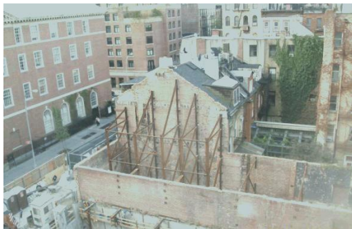
Figure 24: Shows Temporary Structural Steel Bracing
