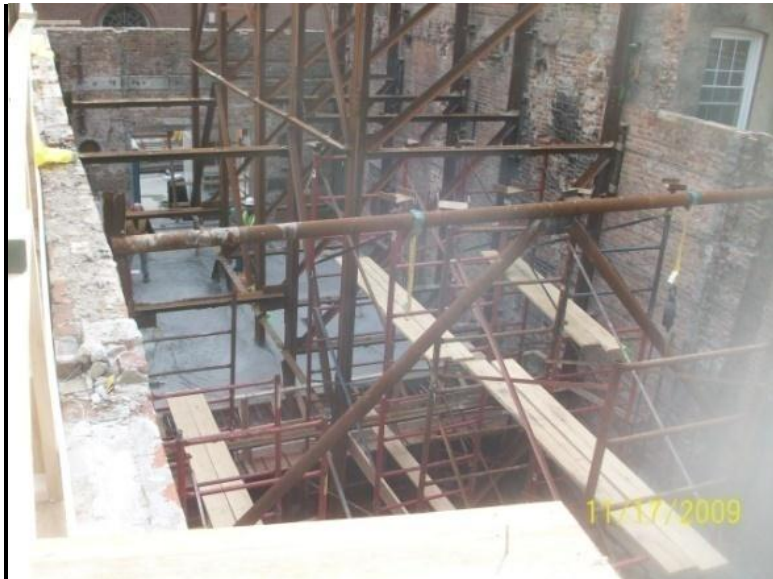
Figure 5: Shows Congested Site Due to Structural Steel Bracing
